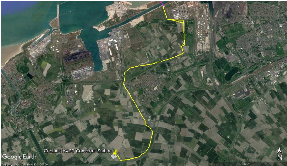
Figure 14 Underground Cable Route in Dunkerque
