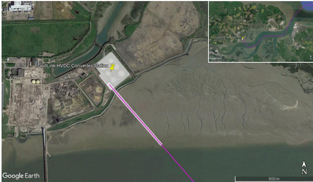
Figure 20 Horizontal Directional Drilling (HDD) of Shore Crossing at Kingsnorth
